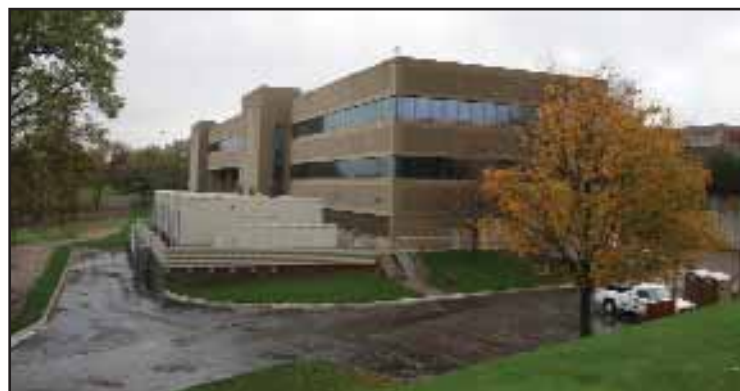
Unysis's renovated facility in Eagan, Minn., sets a benchmark for green data center design.
